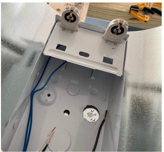
7) Using the largest stepped bit in the set, drill out the hole to ½ inch or a step up to fit the wire connector. Drill from both sides to ensure clean edges.
