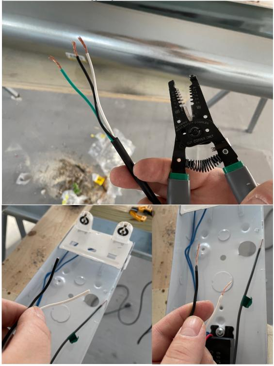
6) Insert the light assembly into the duct. Leave about 2.5-3 inches between the end of the duct and the light assembly. Use the side that has a clean edge. We will use the crimped side to attached the louvered vent assembly. Ensure that the light assembly is straight on in the duct. Then, using a 5/8ths inch drill bit, drill a pilot hole in the center of the knockout to mark the position of where the stepped bit will be used to enlarge the hole.
