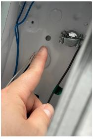
10) Now that the fixture is anchored in on one end, use the same drill bit and do the same thing on the other end of the fixture to lock the fixture into position.
