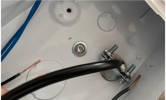
12) Some of the light kits may not come with a ground wire. If they don't do not worry. Strip a wire back and use it as the ground wire. Make sure you keep track of which wire you make the ground wire. You will need to attach this ground wire to the green wire that you stripped earlier. A good idea is to use some green tape.
