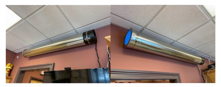
Component cost: Approx 150-160 USD as of 1/27/2021 (excludes tools/fasteners) Air volumes treated: 265-280 CFM on 100% with louvered baffle in place; 380-410 CFM without baffle in place. Note: Using a louvered baffle plate helps to prevent UVC from escaping the tube.
