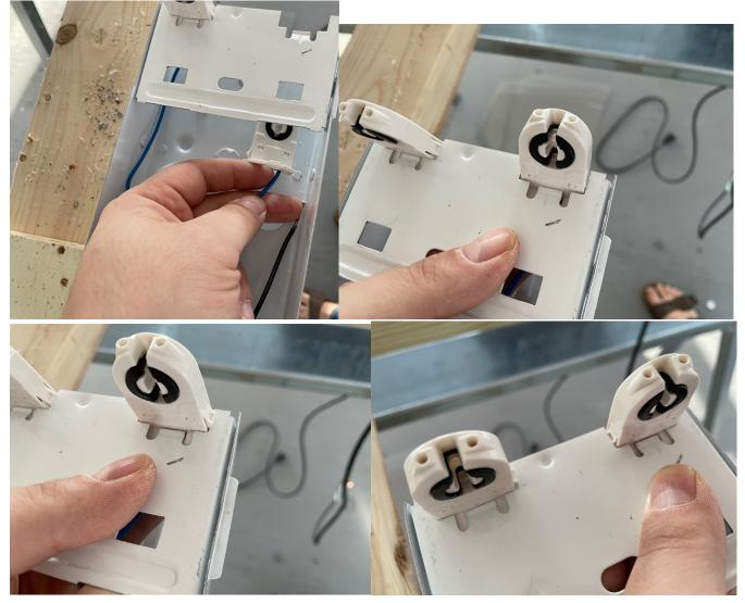
4) Tap the end caps into the light assembly, one on either side
