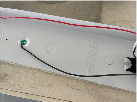
13) Now it's time to join the lighting wires to the stripped wire (the plug lead). Twist the two wires together and then place a wire nut on top. Twist the wire nut until it stops spinning. Do not overtighten. The wire
