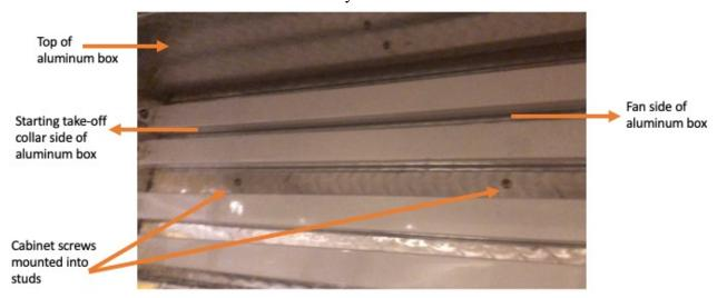
Inside view of the aluminum box. Note, this photo is from an earlier design of the large UVC system when I used 4 individual light fixtures instead of two duplex fixtures. The principal for attaching the aluminum box to the wall, however, is the same.
